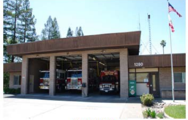
STATION 41 1280 Moraga Way, Moraga
