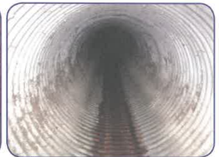
A drainage pipe with the bottom rusted away in comparison to an intact drainage pipe (2015 SDMP)
