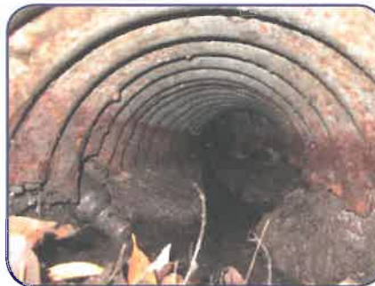
A drainage pipe with the bottom rusted away in comparison to an intact drainage pipe (2015 SDMP)
