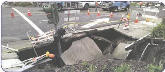
A 30 foot by 15 foot deep sinkhole on Rheem Blvd that developed due to a broken drain pipe on March 13, 2016.
