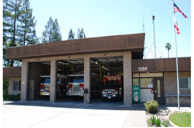
STATION 41 1280 Moraga Way, Moraga
