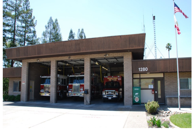
STATION 41 1280 Moraga Way, Moraga
