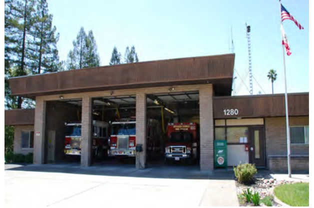
STATION 41 1280 Moraga Way, Moraga
