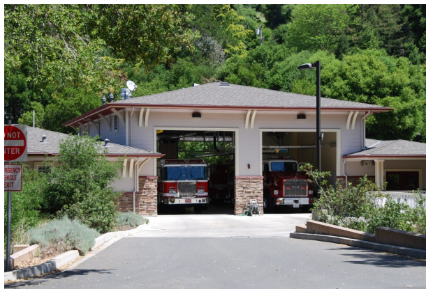
STATION 44 295 Orchard Road, Orinda
