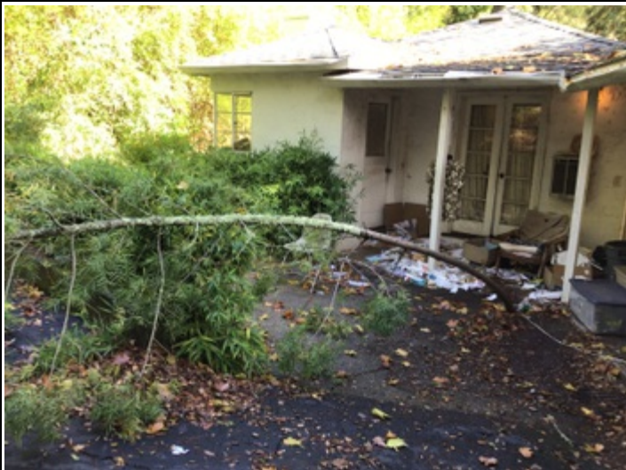
(11/4) Pursuant to our conversation, please complete all the previously mentioned required mitigation by 3/31/2022. Please also remove the new downed tree by the garage and the paper pile by your side door to reduce fire hazard.
