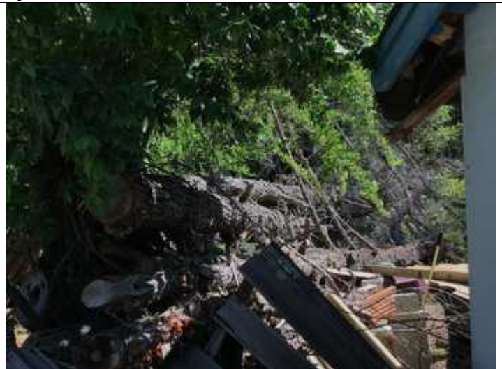
Remove fallen dead trees in back yard.
