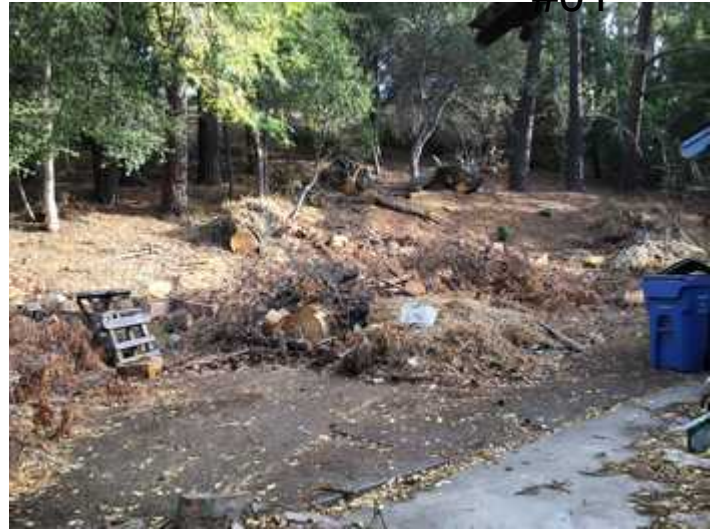
11/6 Please remove all cut tree and tree debris from entire parcel.
