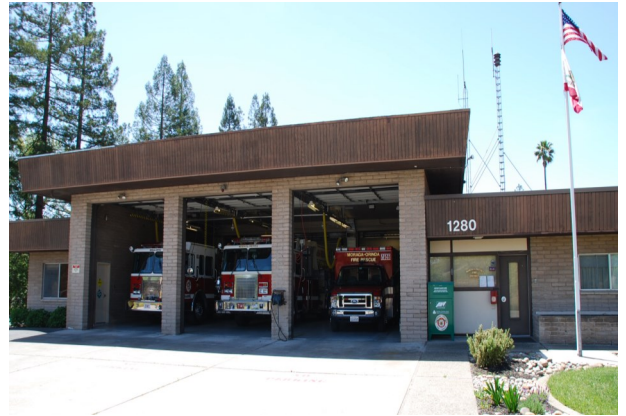
STATION 41 1280 Moraga Way, Moraga
